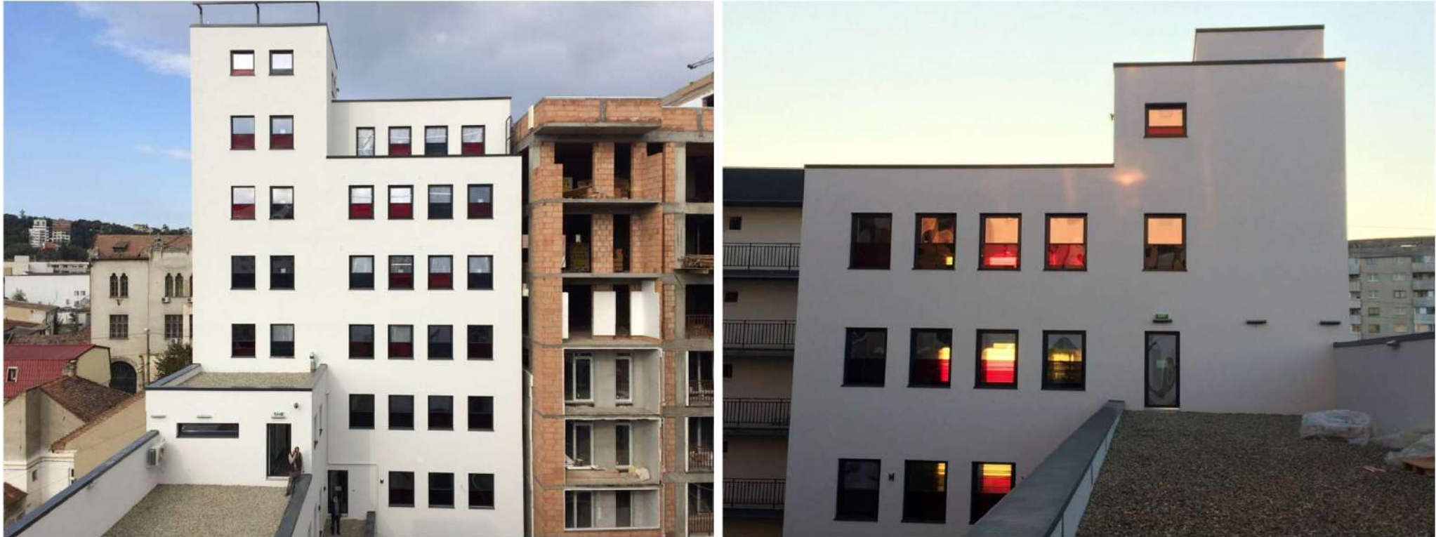
2016 – Stratec BIOMEDICAL, Cluj-Napoca, Romania (Daimler) – I was part of the consultancy team representing the client as project manager for building their office building in Cluj-Napoca
