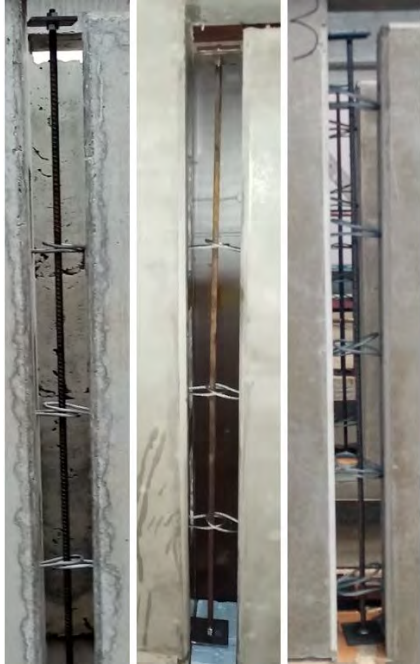
Figure 5-10 Joints before casting (WL1, WL2 and WL3)
