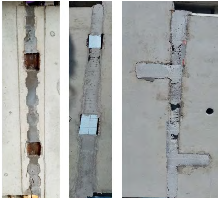
Figure 5-7 Test specimens after grouting (SA1, SA2, SA3)
