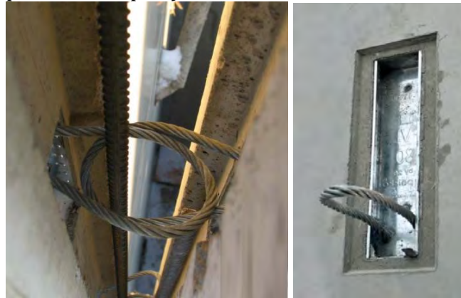
Figure 1-23 Wire-loop connection [30]
