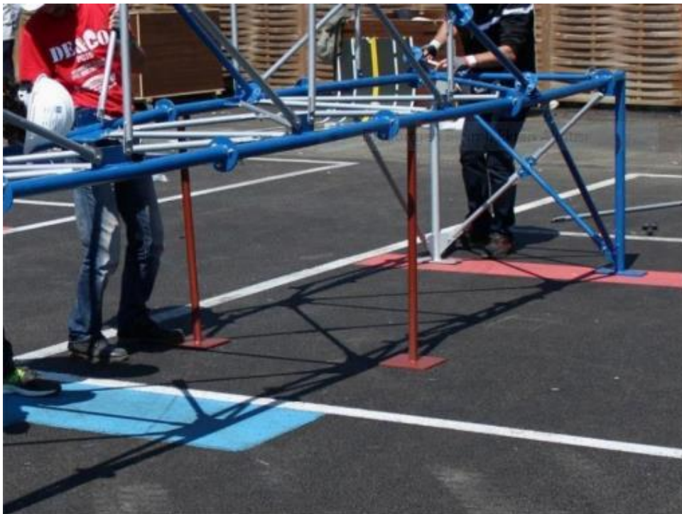
Figure #1: Temporary Support Members (brown painted elements.)
