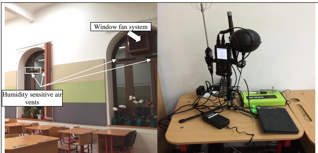
Figure 1. a) Classroom photo with the ventilation systems (humidity sensitive air vents and window fan) and b) Equipment used during experimental campaign
