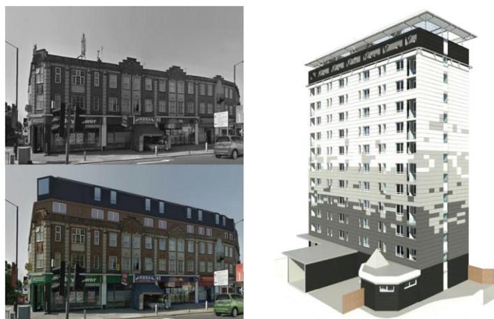
Figure 3. Over-roofing and over-cladding renovations: (a) Italy; (b) Newport City homes [4] Although in Romania, in the last decade, a lot of standards and guidelines concerning the structural, technological and energetic efficiency for these interventions have been elaborated, some aspects
