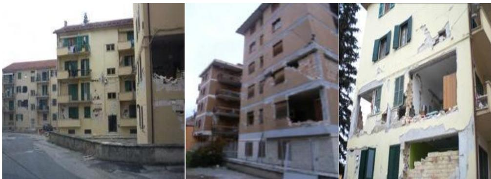
Figure 1. Examples of in-plane and out-of-plane seismic damage to clay unit masonry infill walls.
