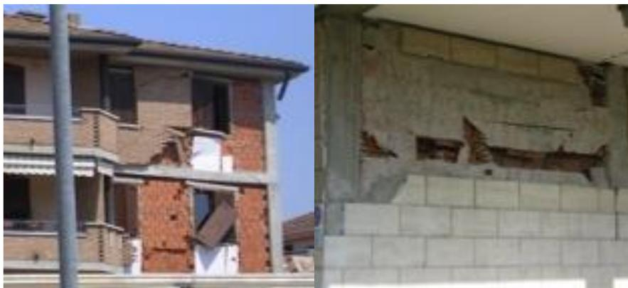
Figure 4. Masonry infill and veneer damage after the earthquake from Emilia, Italy.
