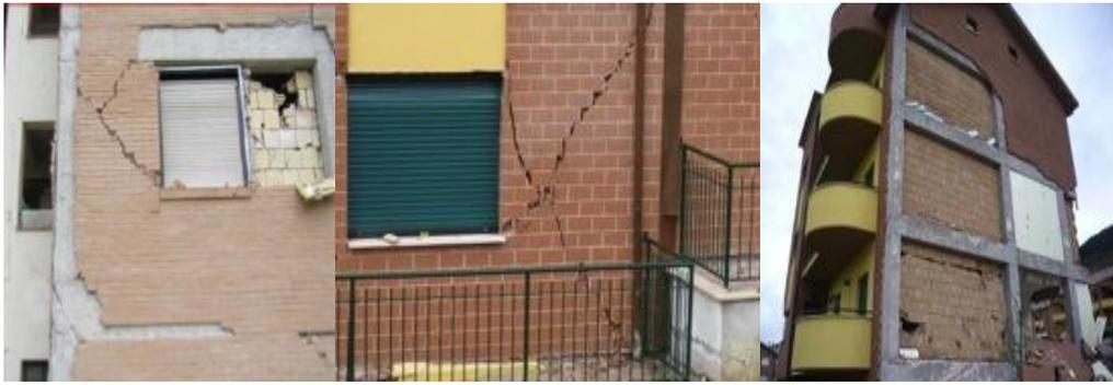
Figure 2. Examples of in-plane and out-of-plane seismic damage to clay unit masonry veneers.
