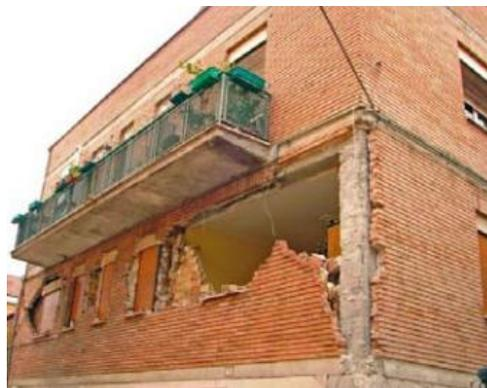
Figure 3. Typical damage of infill wall after the L'Aquila, Italy earthquake.
