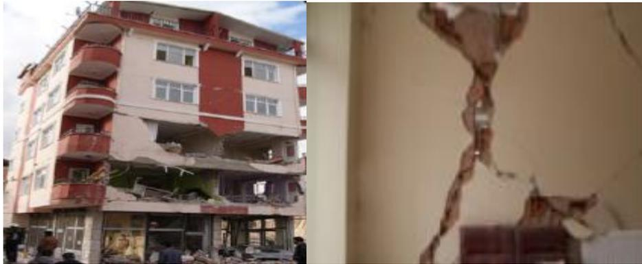
Figure 5. In-plane and out-of-plane failure of masonry infills after the Van, Turkey earthquake.
