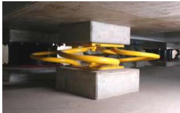
Fig. 2. – Spiral steel damper [3,7]
