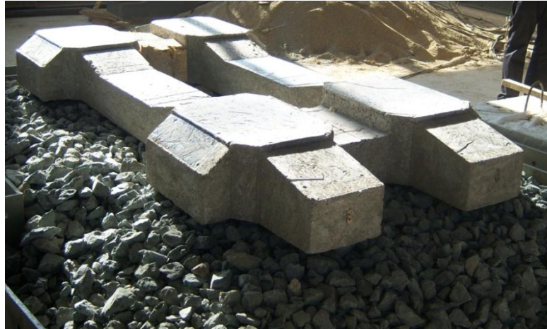
Fig 5. The sleeper placed on the ballast bed
